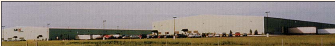
TWO IDENTICAL SIDE-BY-SIDE BUILDINGS Each with 200,000 sq. ft. and 32 loading dock doors
